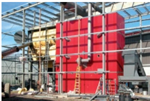
Installation of an 8000 kW boiler
